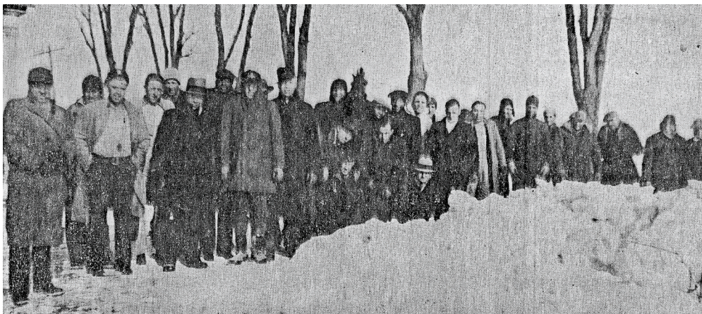
Fig. 91. Further west along National Avenue, travelers became mired in the drifts of the 1936 blizzard. These 31 men sought, and were granted, refuge at the Christopherson farm near New Berlin's western border. They were stranded for three days and two nights before the road was opened sufficiently to proceed. Mrs. Christopherson, with a neighbor's help, provided food and lodging; in return some men helped with chores since Mr. Christopherson himself was stranded in West Allis. The episode is described in more detail in the text.
